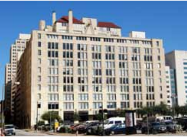
Originally built as a railroad freight warehouse/terminal for the Santa Fe railroad in 1925, this downtown structure was converted into 190 housing units in 1998.
